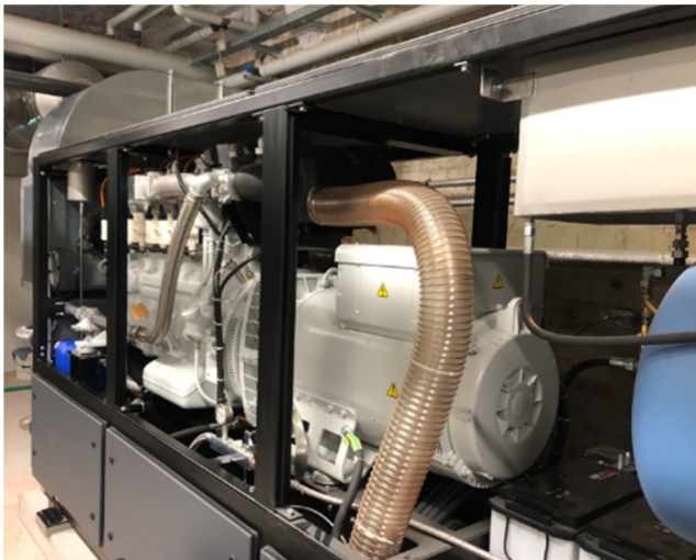
Figure 18: CHP and Boilers of the current heating network of the Baumwollspinnerei, © Cenero Energy GmbH
